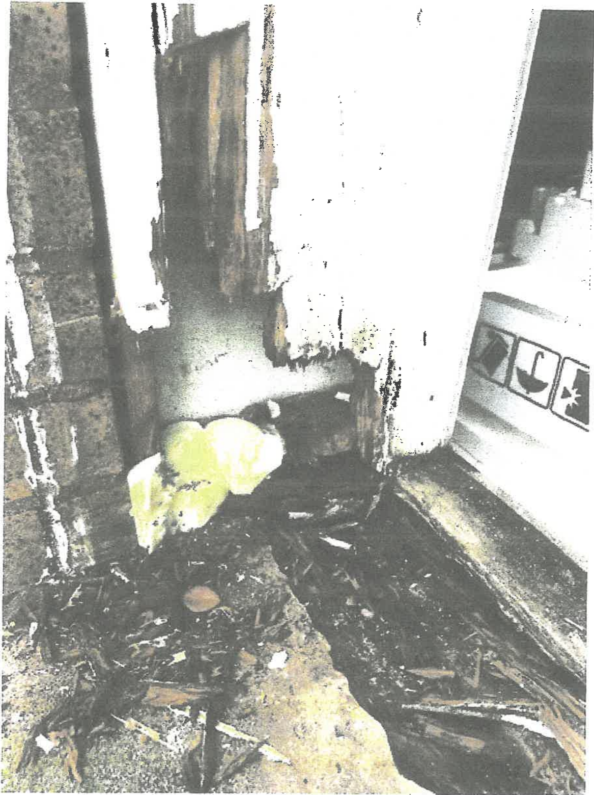
Chase Bowen Rotted Window removed
